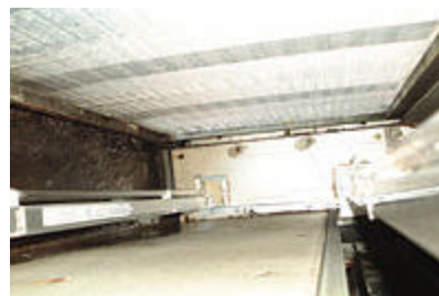
Minimal cuts were made into the unit's
